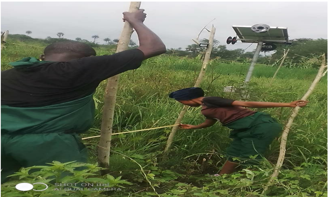
Plate 2: Marking out and pegging on the field.
